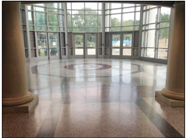
Inside the new dome. See our website for the latest renovation pictures.
